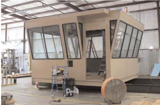
Off-site, factory-built construction is a more controlled, "greener" building process. The centralized construction location also allows for much greater reuse and recycling of materials.
