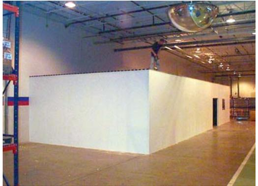
2. Now it's a one-story system with a load bearing roof.
